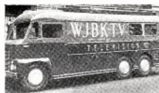
NEW $11,000 TV mobile unit of WJBK-TV Detroit, equipped with RCA two-camera field chain, following WJBK-TV's Oct. 24 premiere, will be used in televising sports and special events. Remote broadcasts will be relayed to TV transmitter by microwave transmitter.
